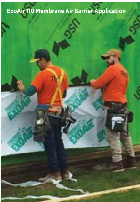
Test Structure Before Securock ExoAir 430 Detailing and ExoAir 110 Application
